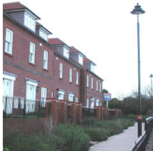
3.4 Front boundary details should not interfere with informal surveillance of the street and must be of robust permanent material such as railings or walls, with or without planting (rather than timber fences).
