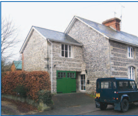
This excellent extension is subordinate to the original house, uses high quality materials and fine detailing.
